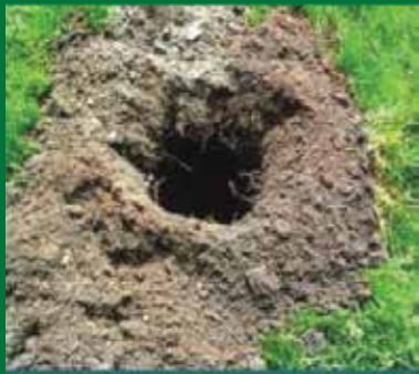
DIGGING THE HOLES
